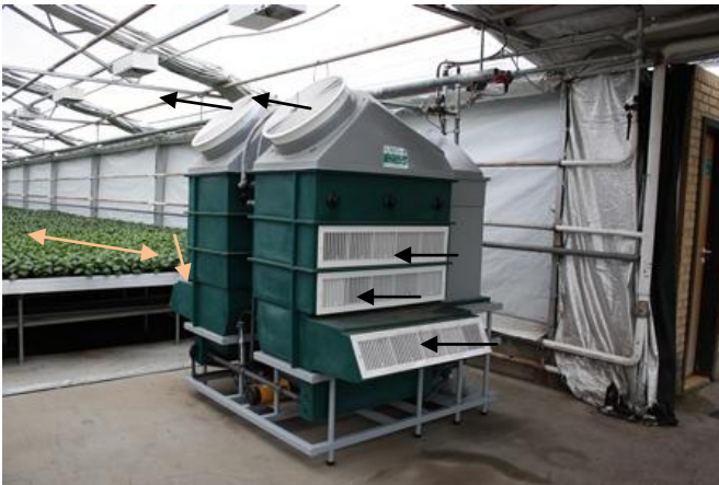
Picture 2. The path taken by air, in spore-trap ventilation unit.
